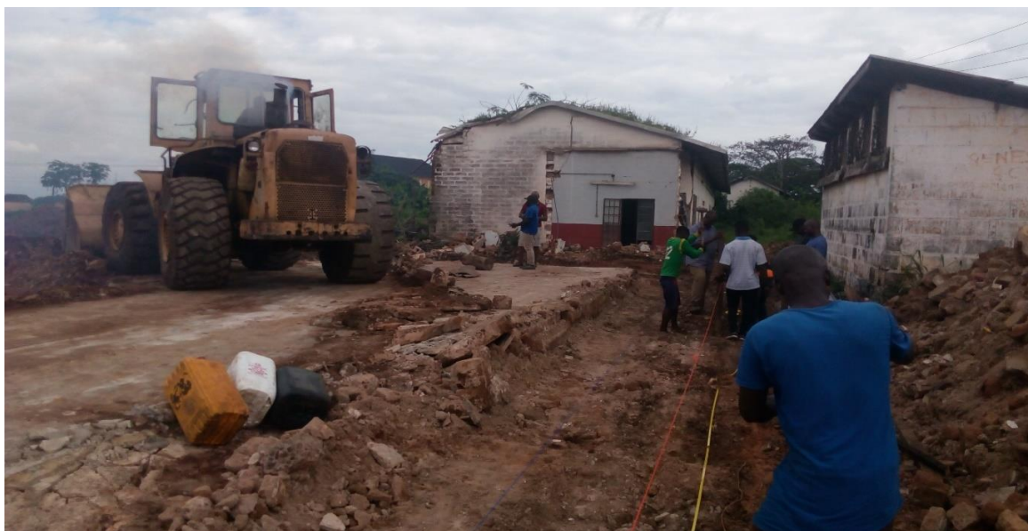
Fig 1. Setting out complete. Excavation in progress
