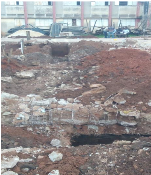
Fig 4 Excavation across for internal partition
