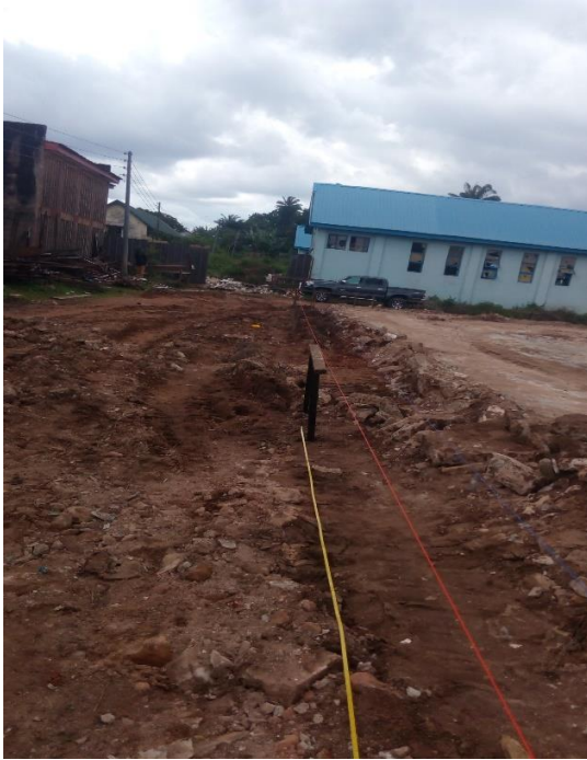
Fig 2 Setting out on the long side complete
