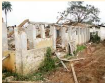
Dining Hall - During demolition
